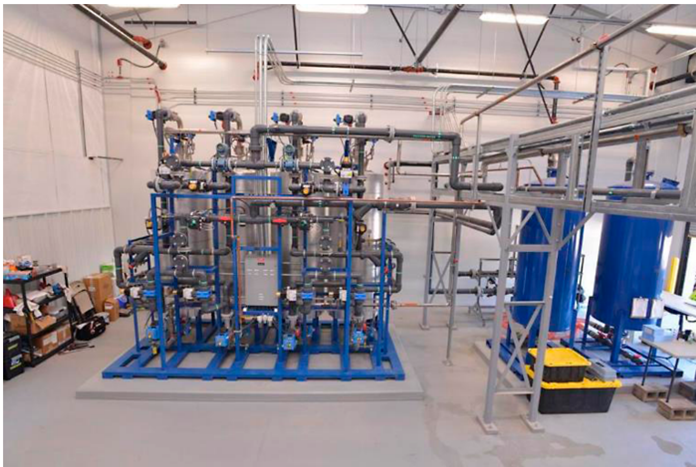
Figure 15-13. Regenerable and polish IX resin vessel skids.
