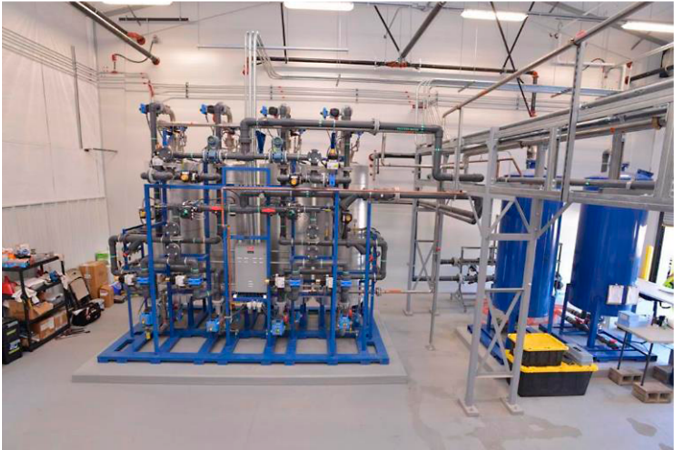
Figure 15-13. Regenerable and polish IX resin vessel skids.
